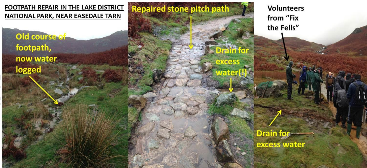
Figure 42 - footpath damage and repair
